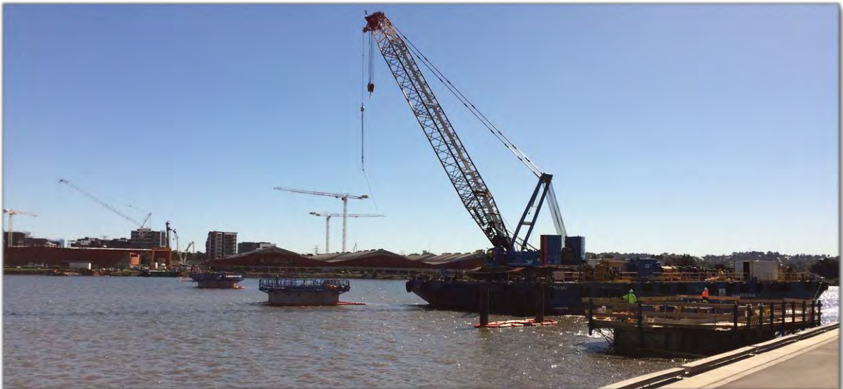
Installation of the bridge foundations in Homebush Bay is now complete
