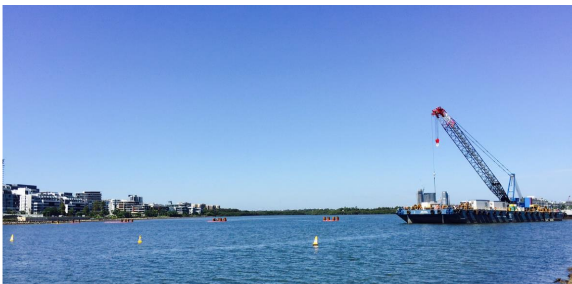
Bridge piling work in Homebush Bay
