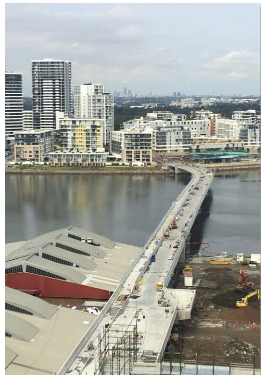
final works on concrete safety barriers
