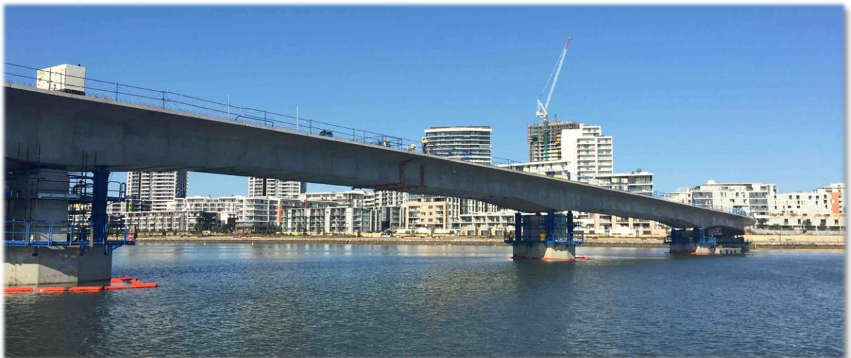
Main bridge deck takes shape - September 2015
